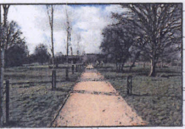
Existing Public Right of Way Re-Aligned To Suit Proposals With Rolling Gravel Finish
